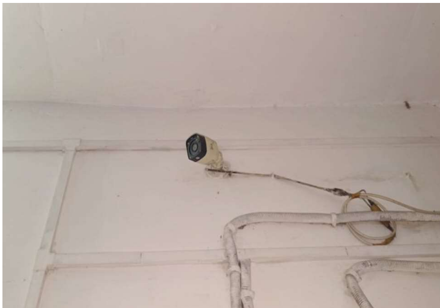
Installation of CCTV camera throughout the campus
