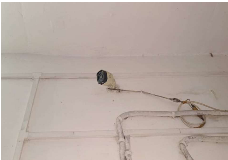
Installation of CCTV camera throughout the campus
